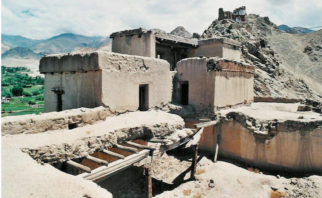
Fig.3. The roof of the Leh palace before its repair by the Archaeological Survey.
